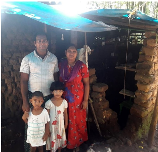
Flood damaged house
